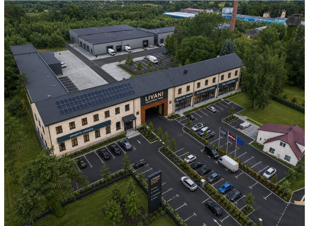
Aerial view: the flagship, solar panels and logistics halls in the yard
